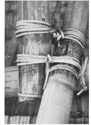
Image 22: Connections using bamboo strips
