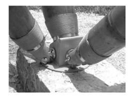
*Image 28: Fixing the canes to the foundation with a metalic profile*
